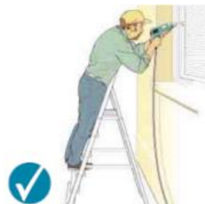
Figure 7b Correct - steps facing work activity
